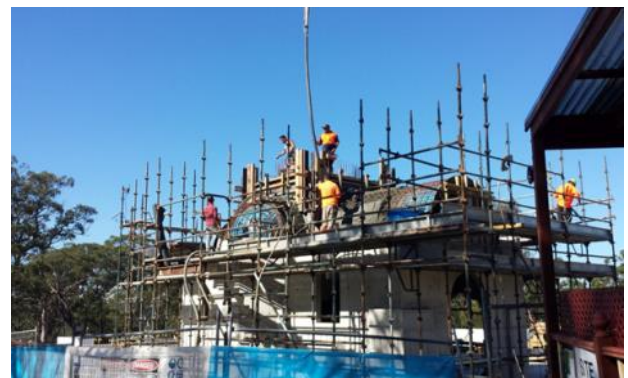
St Irene's chapel during construction
