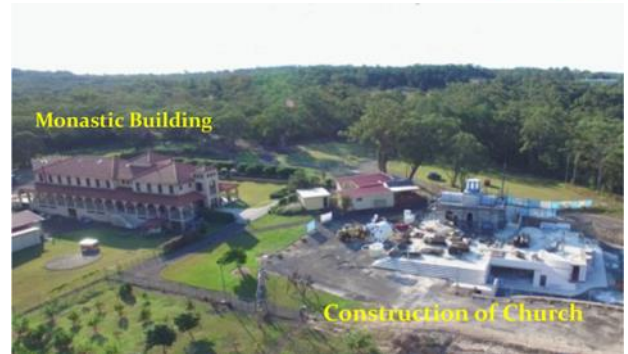
Holy Cross Monastery buildings, with the Katholikon currently under construction
